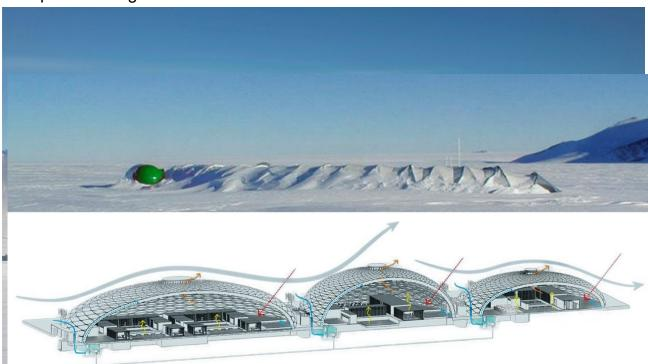
In these adverse weather conditions, architects have come up with ingenious solutions. For instance, the English Halley VI station consists of eight modules, all mounted on hydraulic legs with ski-like mechanisms. This allows the station to be moved quickly and easily with the support of heavy equipment.
